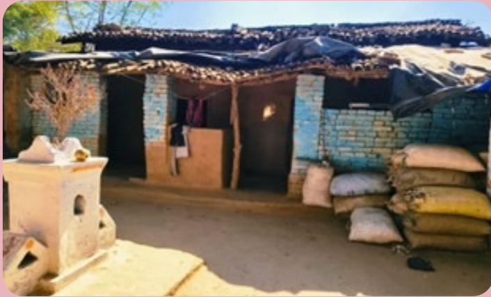
Housing condition >> Mud brick walls with country tile roof
